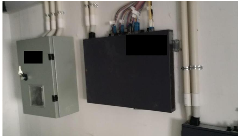
Figure 132: RHUB used for connecting pRRUs in the test network configuration.
