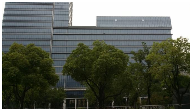
Figure 129: A new office building used for 5G NSA indoor coverage measurements.
